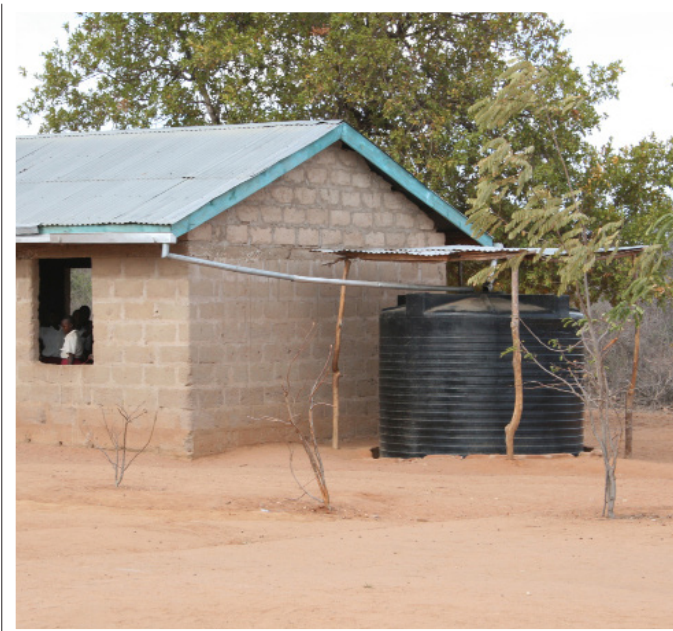
Roof catchment for Primary School in Eastern Mwingi.
