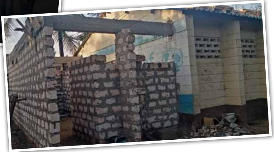
Amani Primary School, Mombasa County - ongoing renovations
